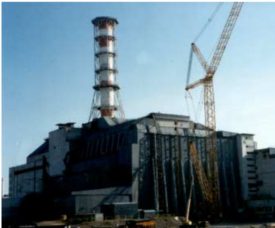
Figure 3: The Chernobyl Nuclear Plant UKRITIYE (shelter).
